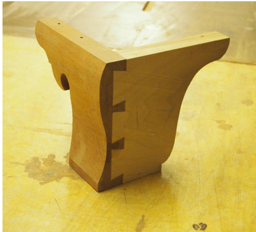
Rear Ogee Bracket and Brace
